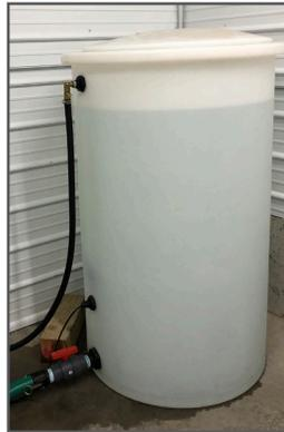
250-gallon holding tank, floats and supply plumbing
